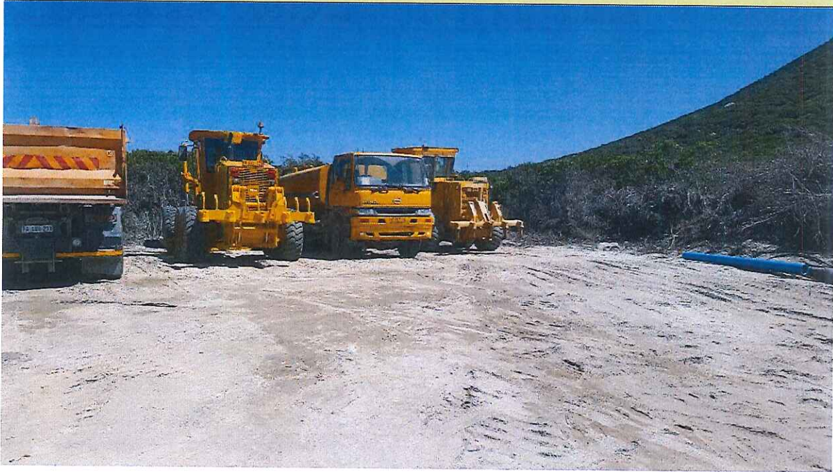
Figure 11: Construction site: Storage area for plant and equipment
