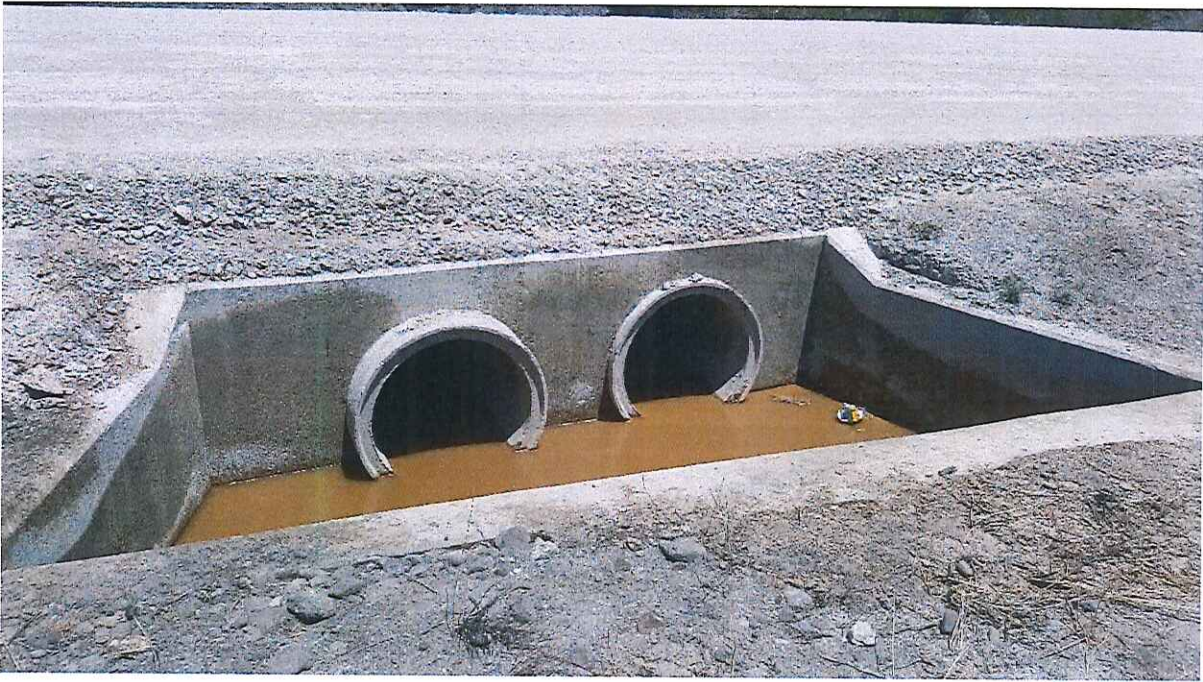
Figure 9: Pipe-culvert inlet after construction
