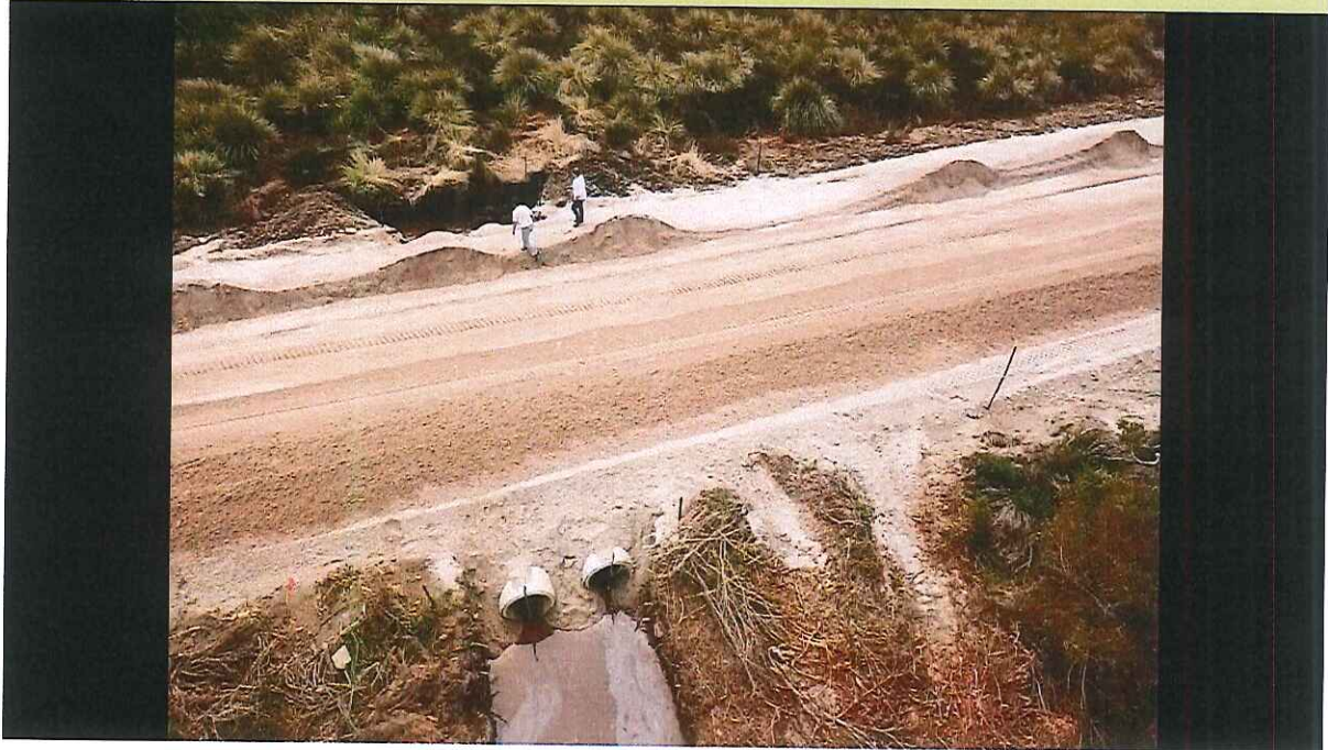
Figure 7: Pipe-culvert at km 6.34 prior to construction
