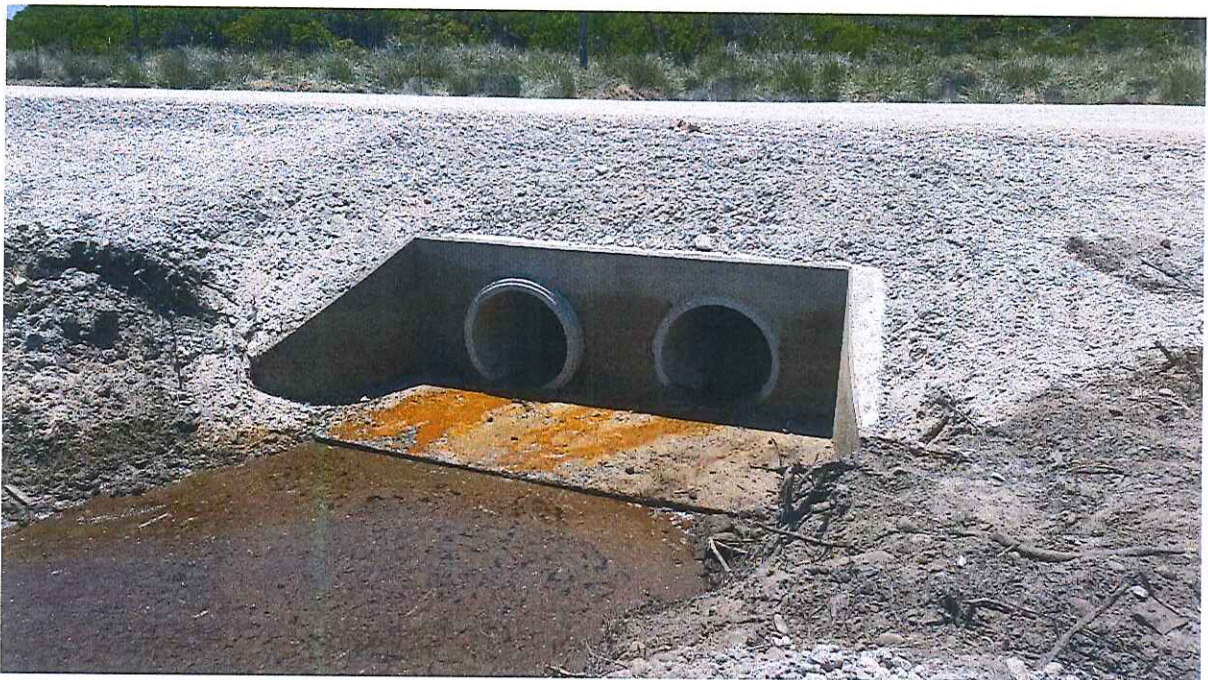
Figure 8: Pipe-culvert outlet after construction
