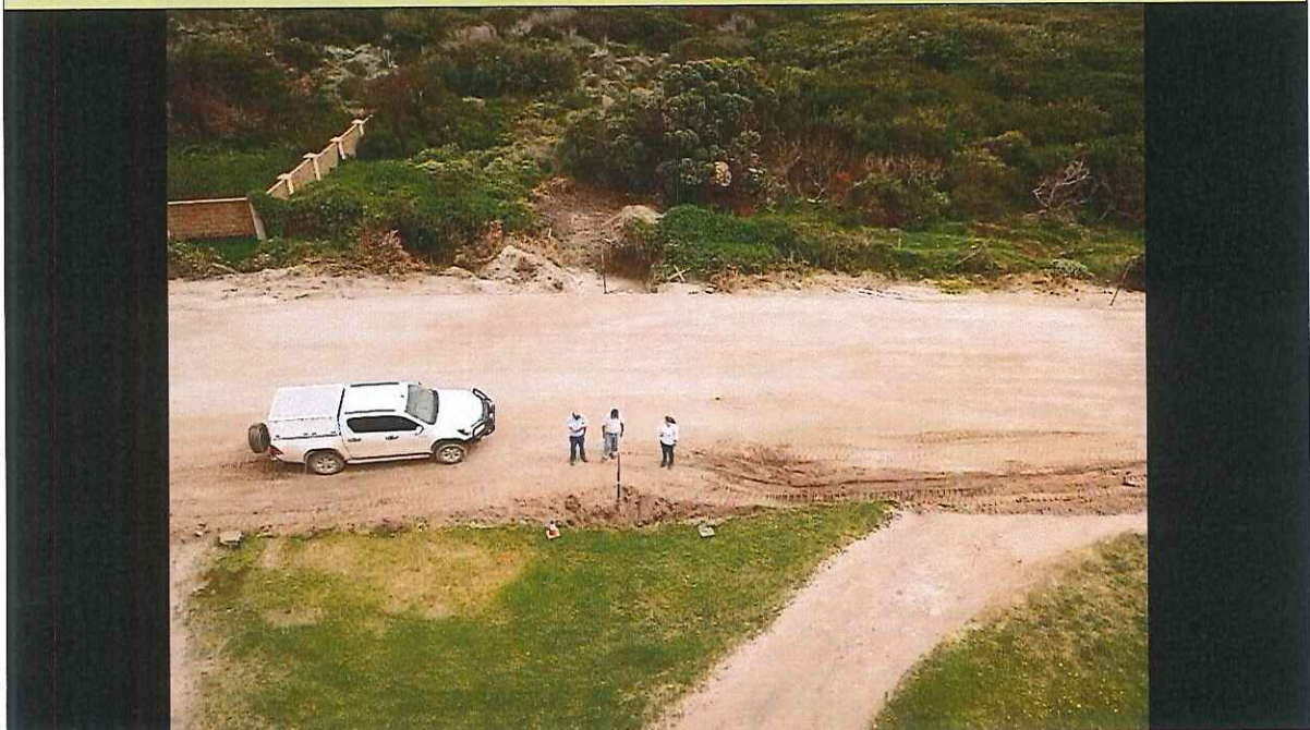
Figure 6: Pipe-culvert at km 5.31
