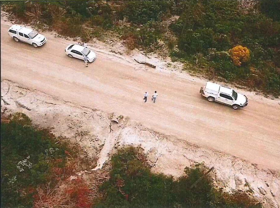
Figure 17: Pipe-culvert at km 7.42
