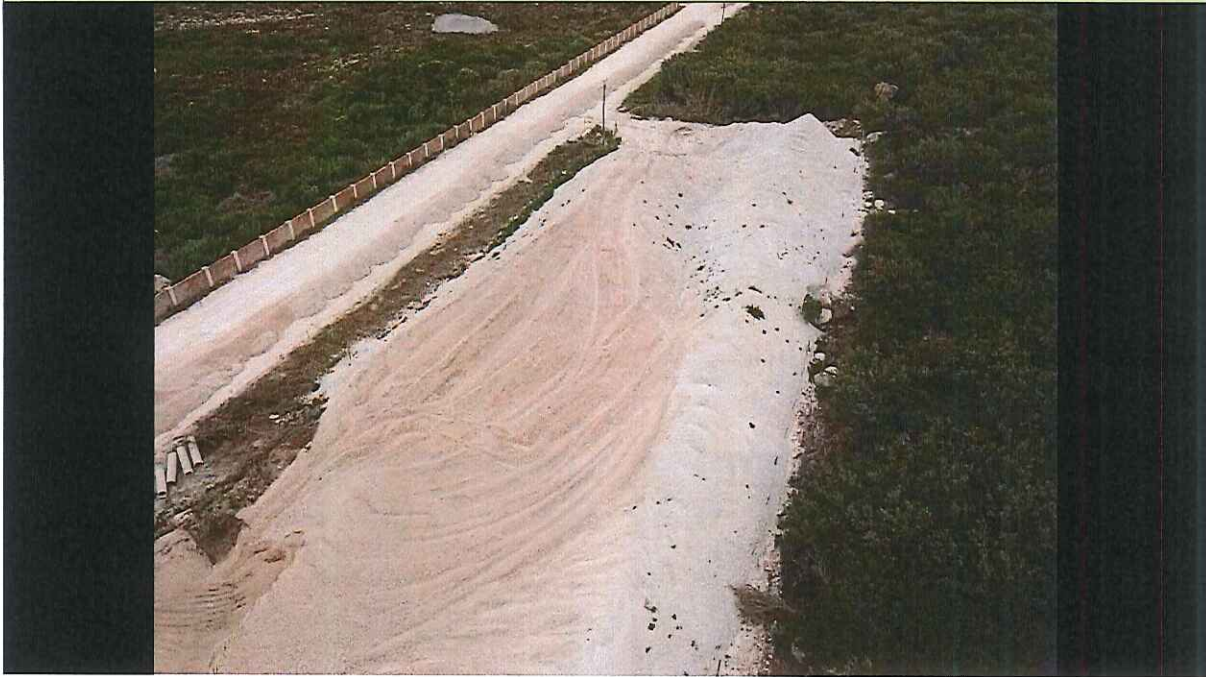
Figure 18: Construction site: Stockpile site
