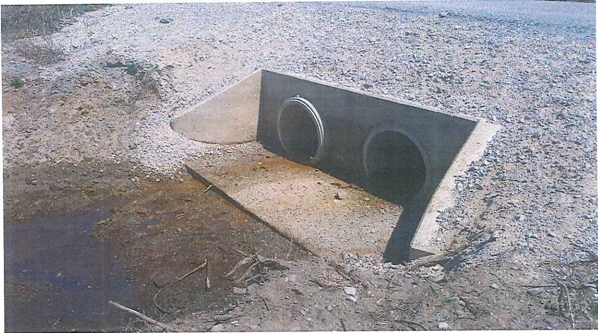
Figure 12: Pipe-culvert outlet after construction
