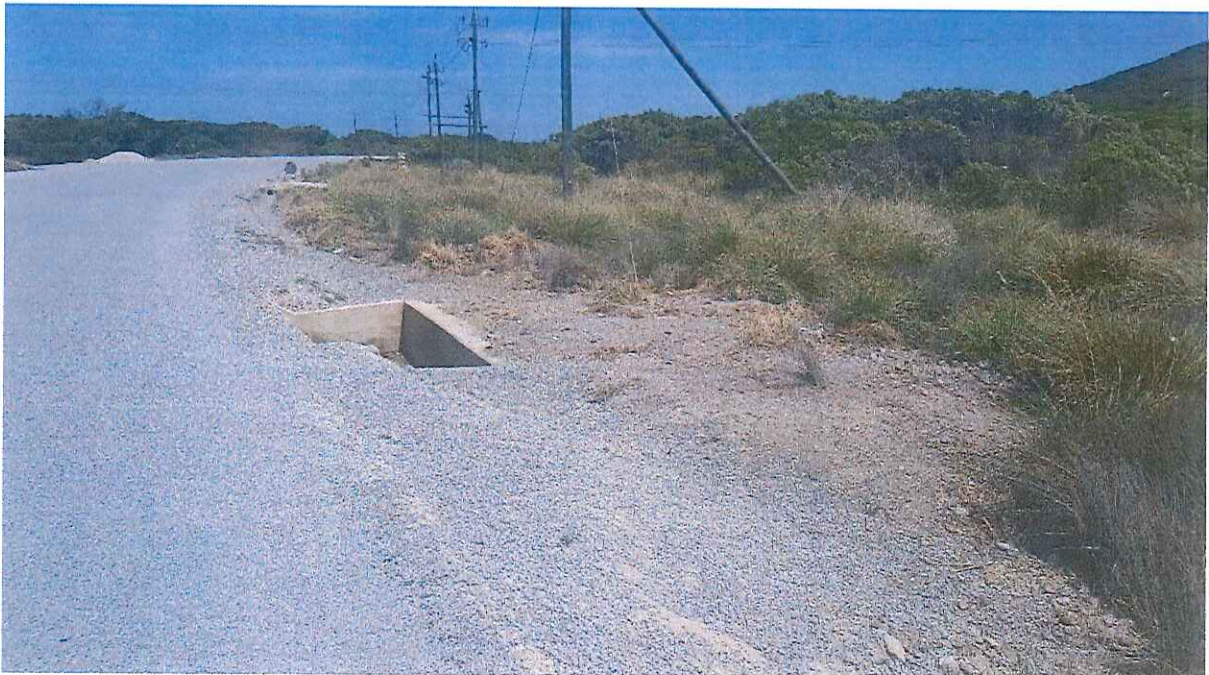
Figure 15: Pipe-culvert inlet after construction prior to rehabilitation
