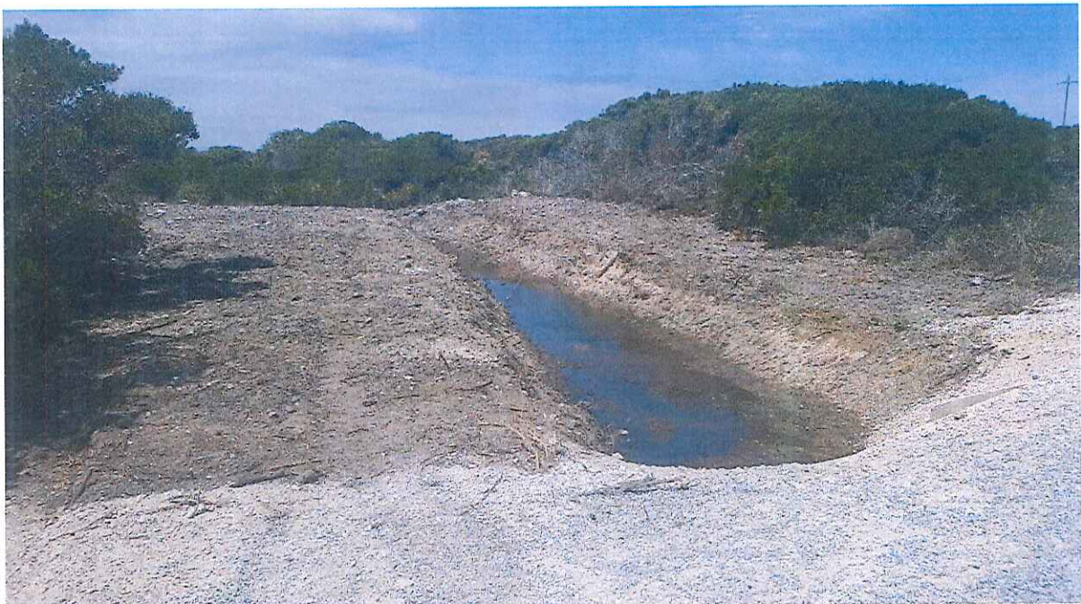
Figure 13: Culvert outlet drainage line.
