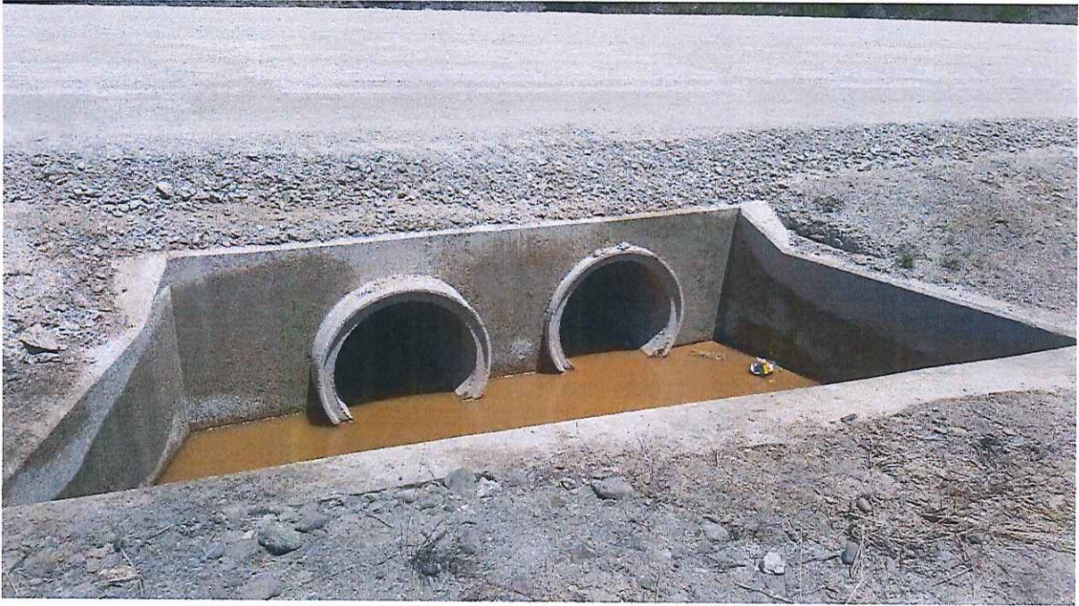
Figure 14: Pipe-culvert inlet after construction
