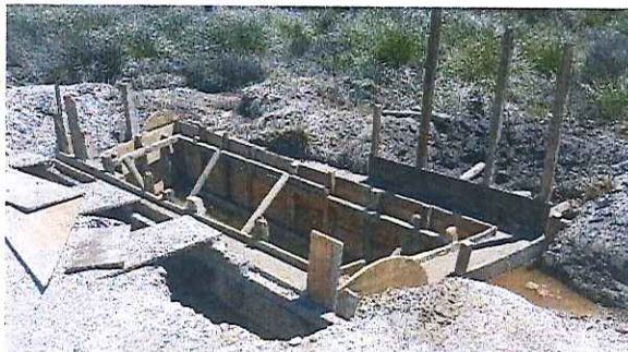
Figure 10: Construction of new culvert inlet
