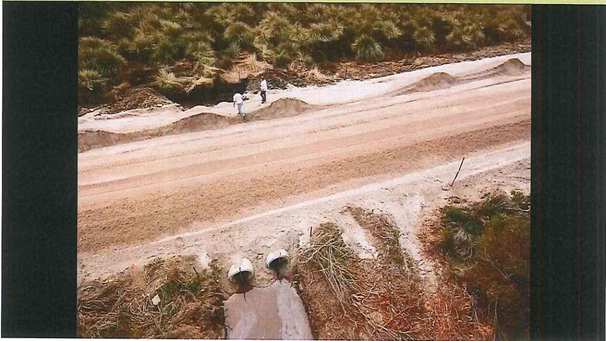
Figure 7: Pipe-culvert at km 6.34 prior to construction
