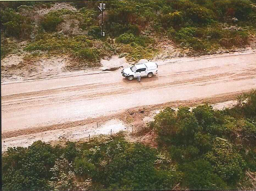
Figure 16: Pipe-culvert at km 7.07
