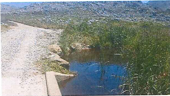
Figure 18: Water abstraction point –09/01/2020
