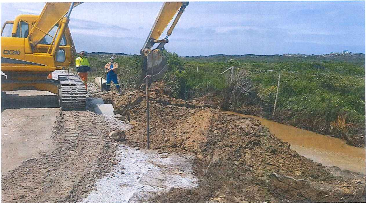
Figure 8: Culvert at km 4.08 outlet during construction
