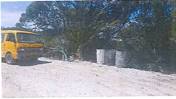
Figure 17: Construction site: Storage area for plant and equipment
