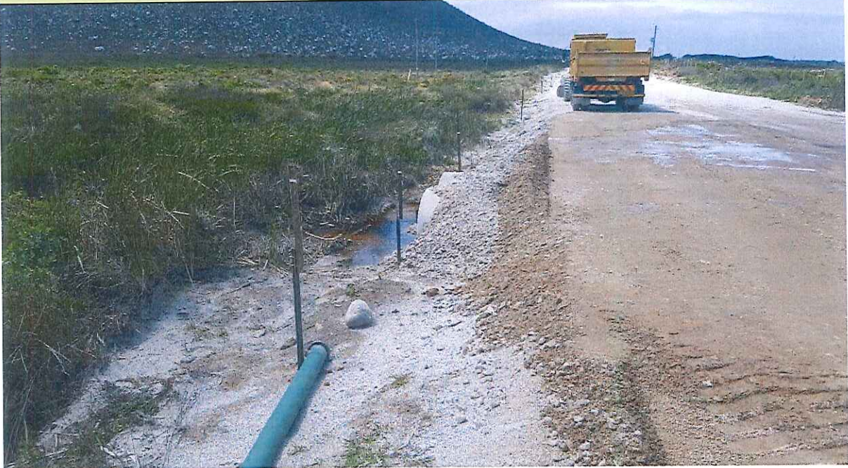
Figure 7: Culvert at km 4.08 inlet after construction.
