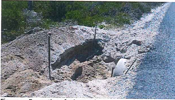
Figure 14: Excavation of culvert at km 7.42
