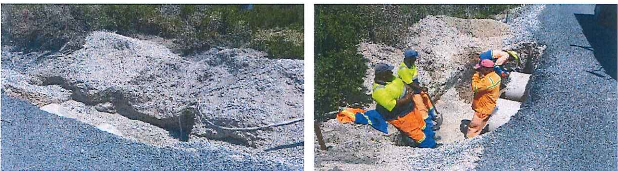
Figure 13: Excavation of culvert at km 7.07
