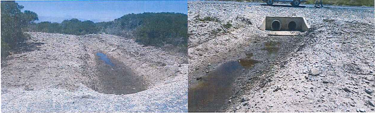
Figure 11: Drainage channel at culvert at km 6.34 outlet
