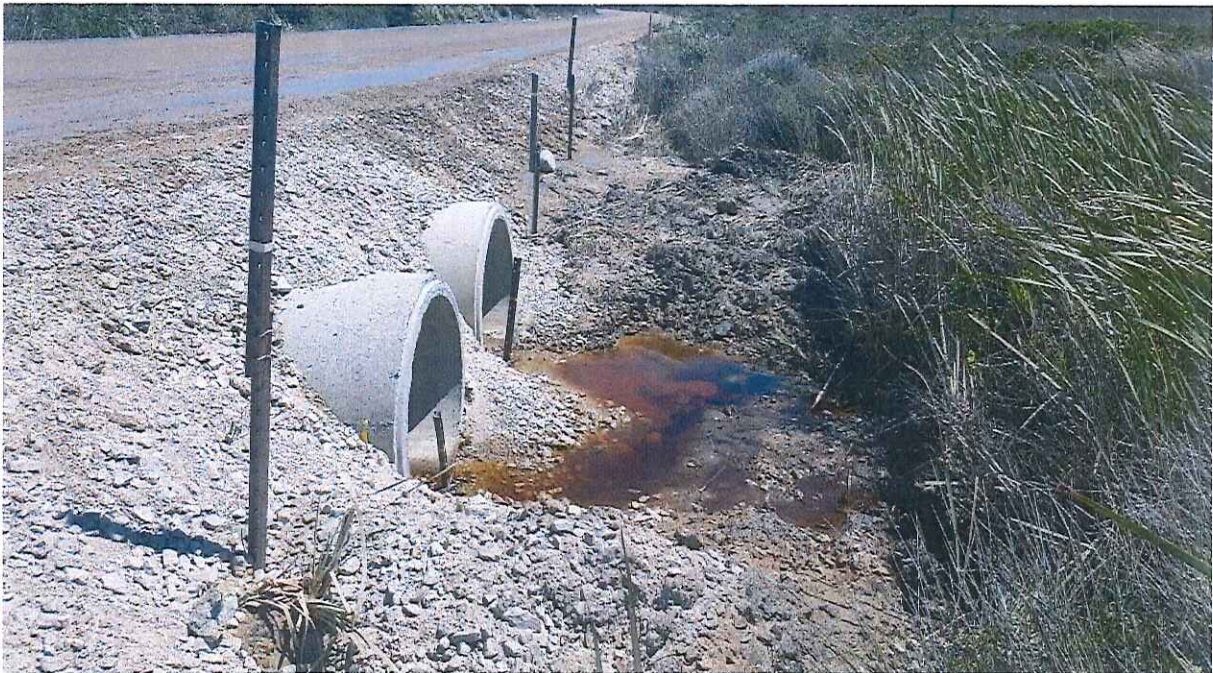
Figure 10: Culvert at km 4.08 outlet after construction.
