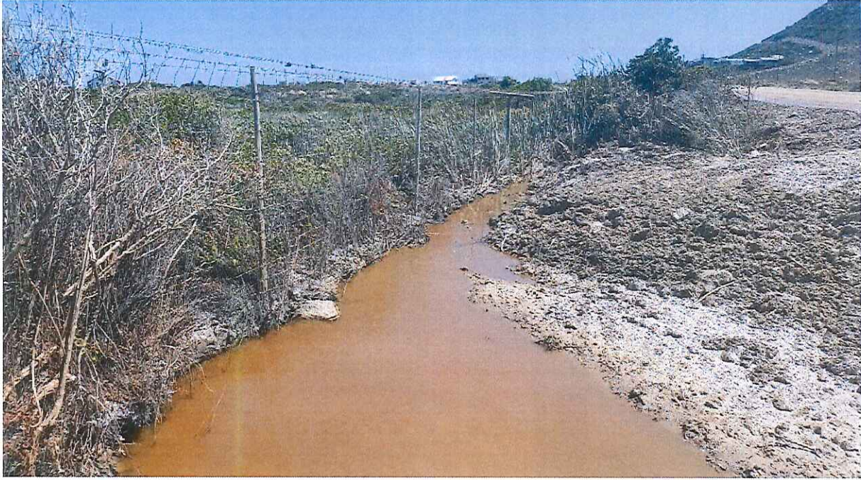
Figure 9: Culvert at km 4.08 outlet - Drainage channel
