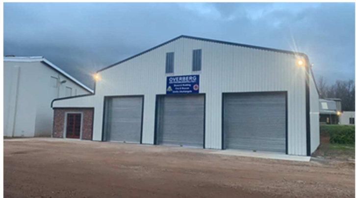
Fire Station at Grabouw
