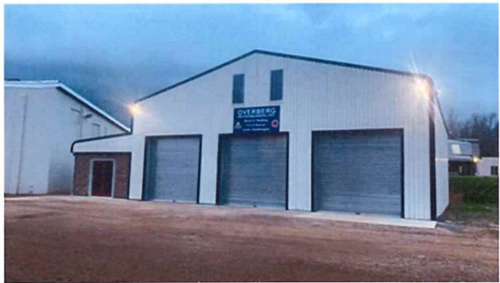
Fire Station at Grabouw
